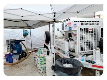
The six-person crew from HiTech used crushed glass and a vapor blaster to prepare the steel surface. They achieved a profile that adhered to the SSPC-SP-6 standard.
